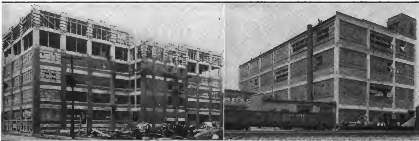
The Hyatt Roller Bearing Co., Newark, N. J., has added a six-story and basement structure, 200 by 75 feet and giving an increase in floorspace of 150,000 square feet
